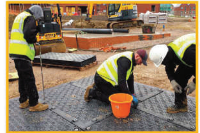
Connect using speed brace or impact wrench
