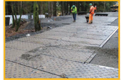
MaxiTrack mats can be half staggered to fit the required space
