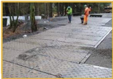
Mats can be half staggered to fit the required space
