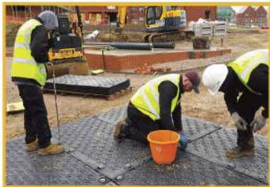
Connect using speed brace or impact wrench
