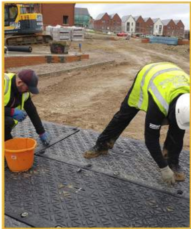
Build trackway uphill if possible
