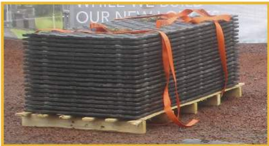
Store pallets on firm level ground
